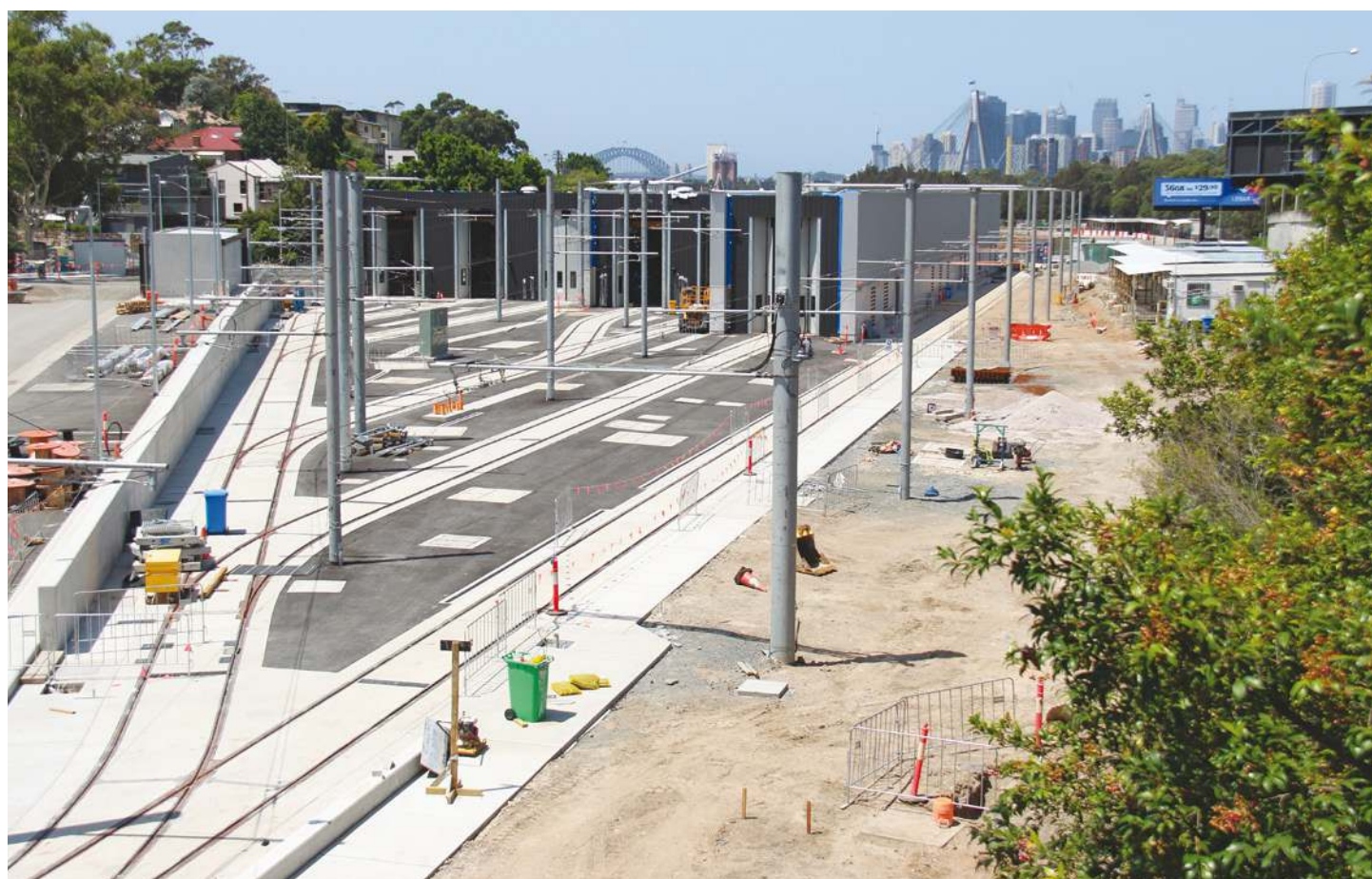
A new tram maintenance facility is being constructed adjacent to the Lilyfield light rail station to service the CBD and South east light rail project. The new facility is located on part of the former Rozelle rail goods yard and it will be able to provide heavy maintenance on up to six trams at one time from the fleet of 60 Alstom Citadis XO5 trams which will be based at Randwick. A substation adjacent to the facility was opened last August. This Saturday, 26 January 2019 view shows the maintenance facility with the Sydney CBD and Harbour Bridge forming the backdrop. John Hoyle
