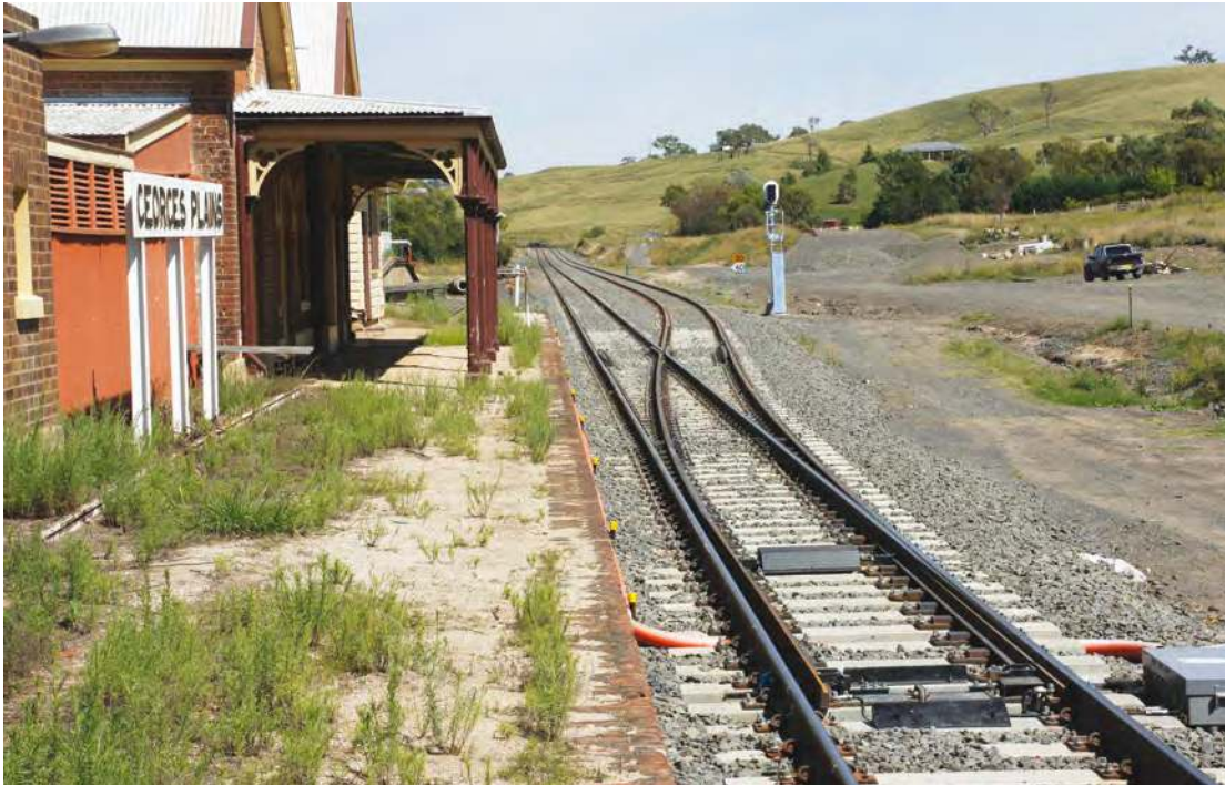
The eastern end of the new Georges Plains crossing loop is located adjacent to the increasingly decrepit railway station. In line with an increasingly common practice, concrete bearers are used for the pointwork. The new Up Loop Starter signal (GP 6) is in the background. Lawrance Ryan
