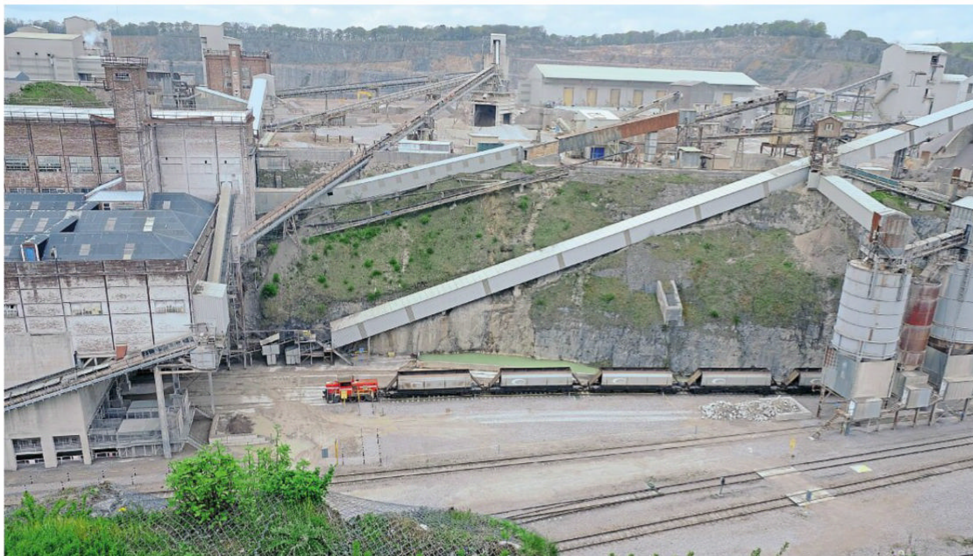
Above: A network of conveyors link the various limestone processing and cement plants, with the loading hoppers set deep within Great Rocks Dale. Viewed from this height, the sheer scale of the operation makes full-size trains look like 'N' gauge models! BEN JONES
