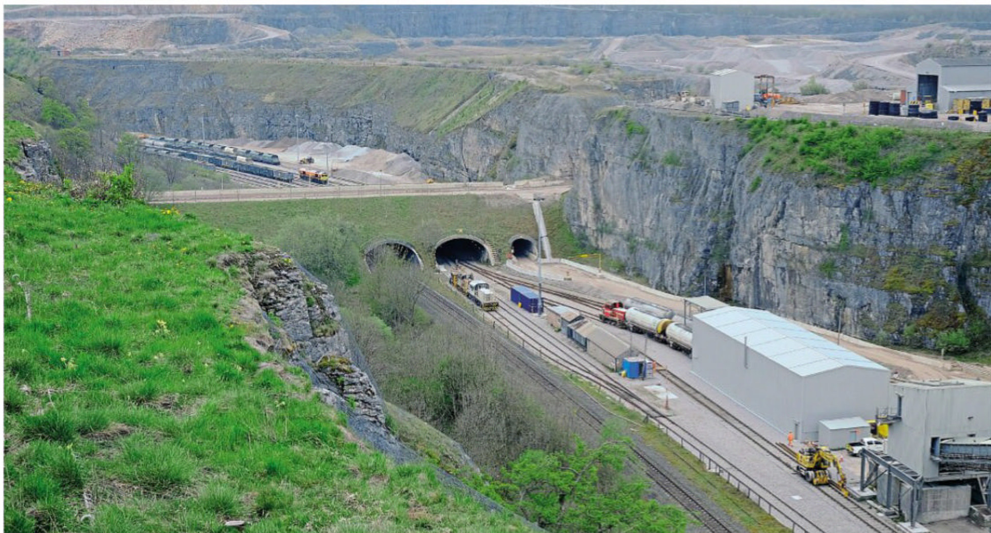
The southern and central parts of the rail sidings are separated by the road embankment linking Tunstead and Old Moor quarries. This view shows the wall loading sidings, where wagons are loaded manually by mechanical shovels. Closer to the camera is one of the cement loading buildings, with High Peak and Dovedale visible in the centre. BEN JONES
